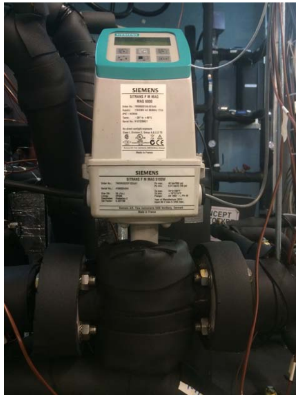
Fig. 3.4- Magnetic SITRANS FM MAG5100 W
