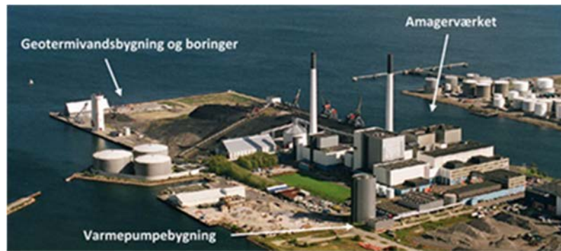
Figure 1.2– The geothermal plant in Amager [4]
