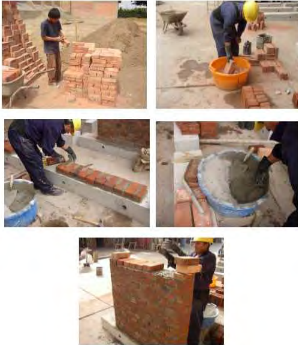
Fig. 2.9 – Panels construction process
