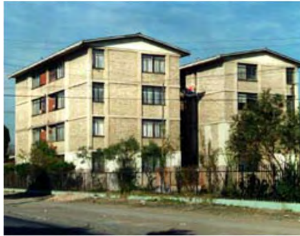
Fig. 1.12 - Confined masonry housing
