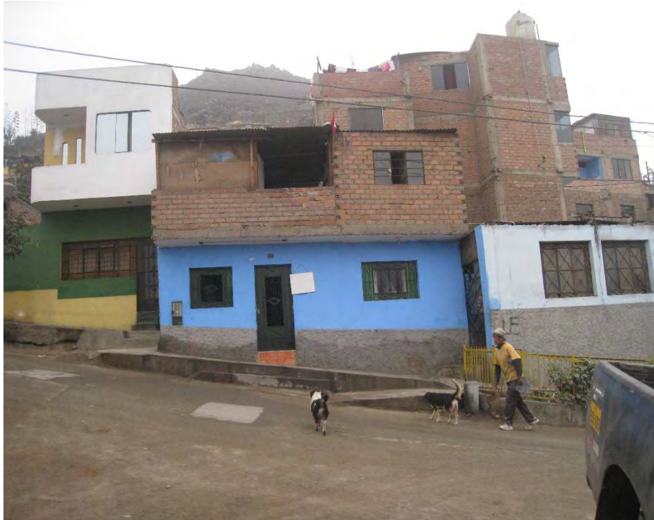
Fig. 3.5 – House with plastered and painted facade at first floor and exposed brick at second floor
