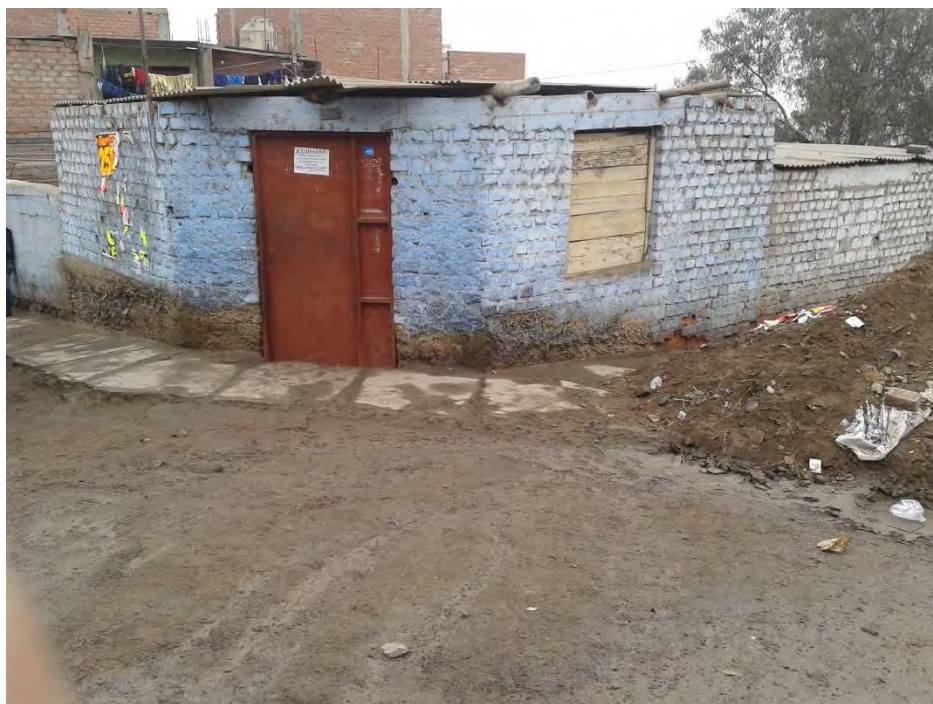
Fig. 3.6 – House with just painted facade
