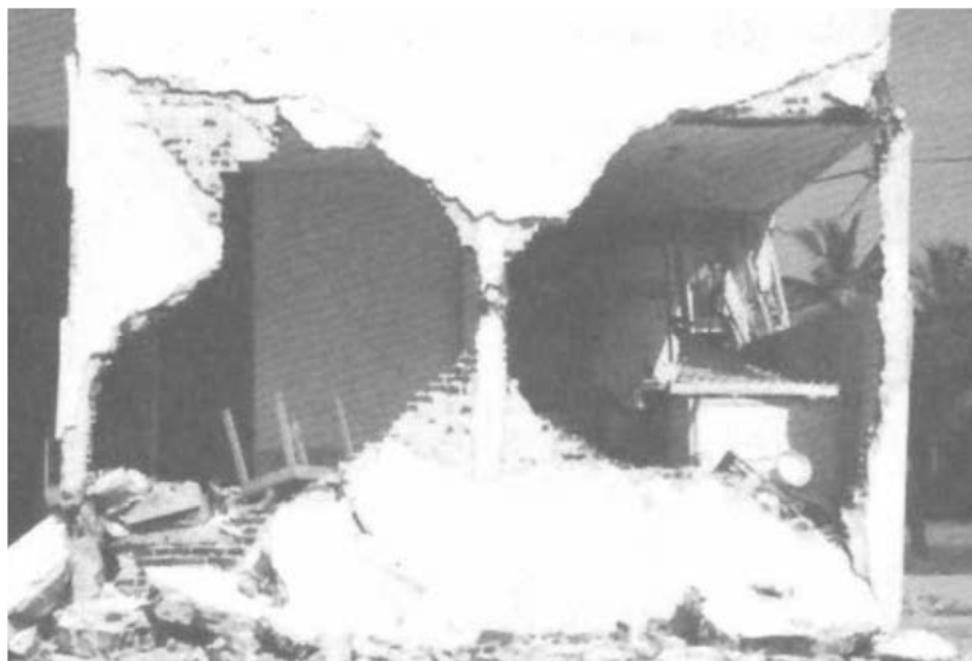
Fig. 1.16 - Damage to confined masonry construction in the 1985 Llole, Chile Earthquake
