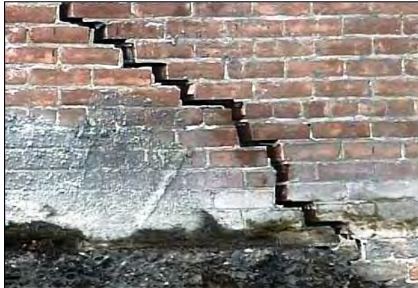
Fig. 1.20 – Brittleness of mortar
