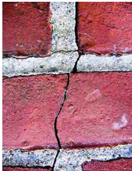
Fig.1.21 – Brittleness of cored bricks
