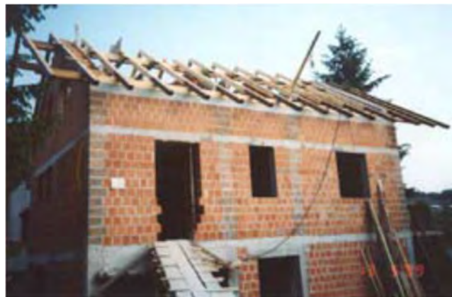
Fig. 1.15 - Confined masonry housing during construction
