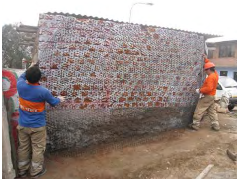
Fig. 3.2 – Reinforcement of part of a house
