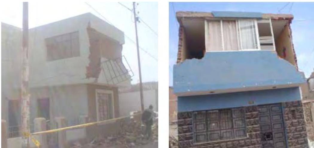
Fig. 3.9 – Seismic effects in unconfined walls
