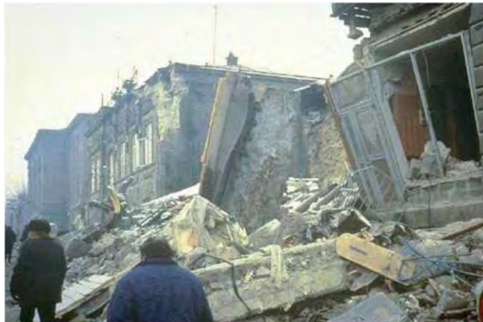
Fig. 1.9 - Collapse of brick masonry buildings in the 1988 Spitak earthquake
