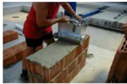
c) Thin layer joints
