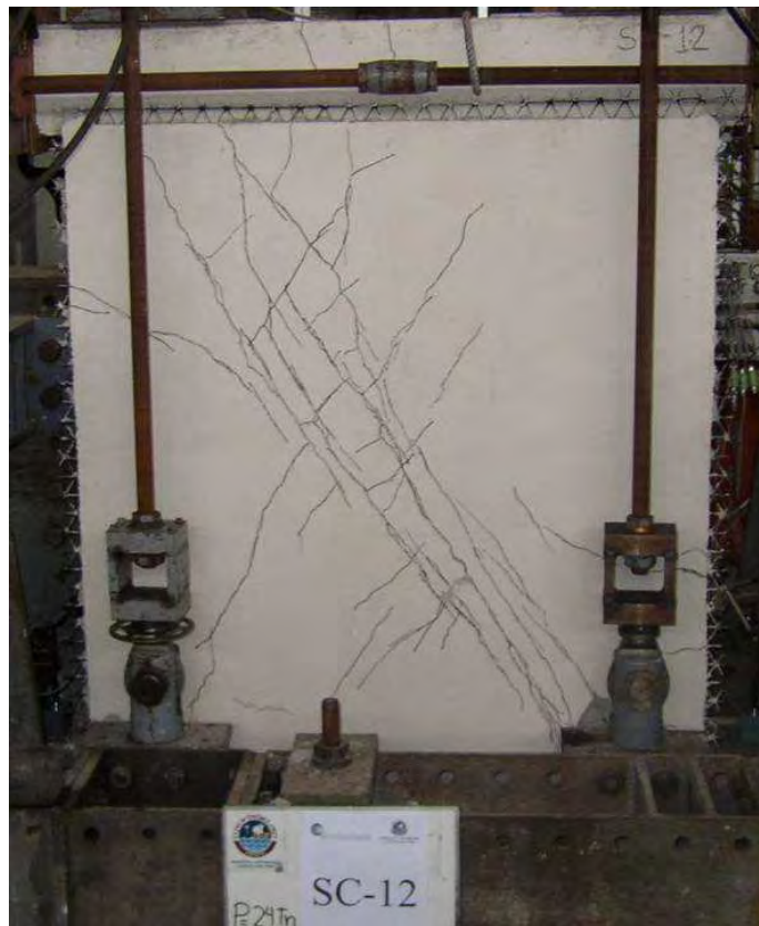
Fig. 2.30 – Cracks formed during the shear – compression test
