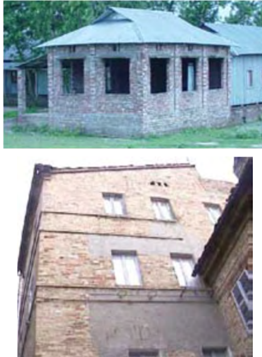
Fig. 1.4 - One and four story unreinforced brick masonry
