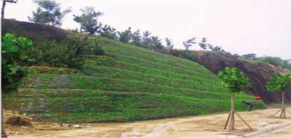
Figure 1.14. Slope stabilization with vegetation (Portar, 2008)
