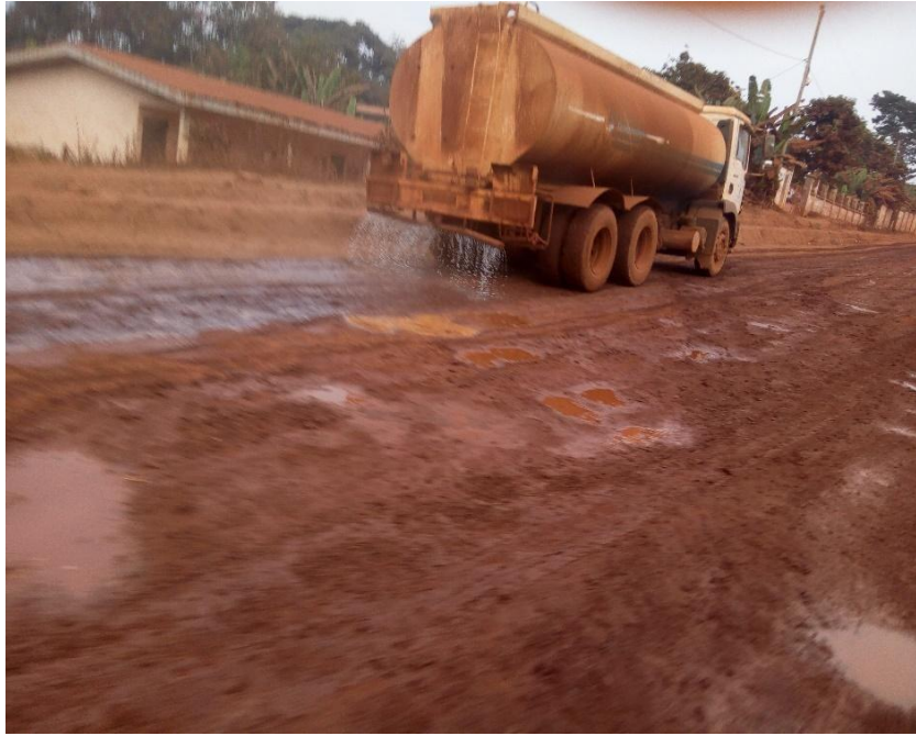
Fig 13: Watering of site against dust pollution
