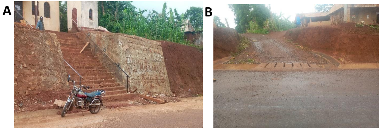
Fig 12:A) Staircase and masonry walls for stabilization; B)slabs to access homes
