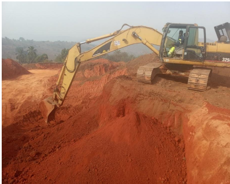
Fig 16: Borrow pit exploitation
