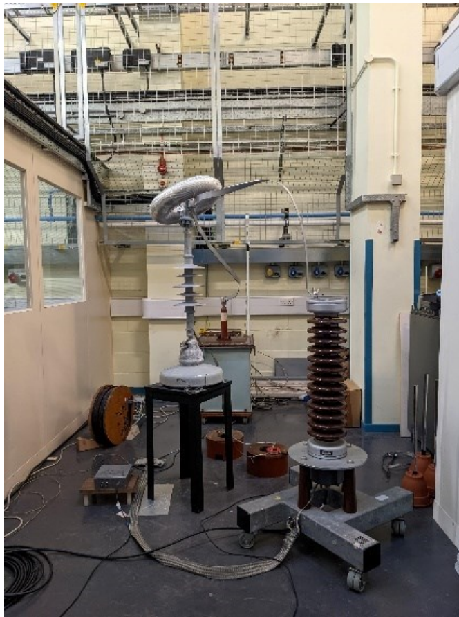
Figure 3.16. Final measurement setup for the insulator tests.
