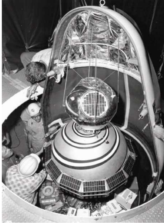
Figure 1.1: Transit 2A during launch preparations
