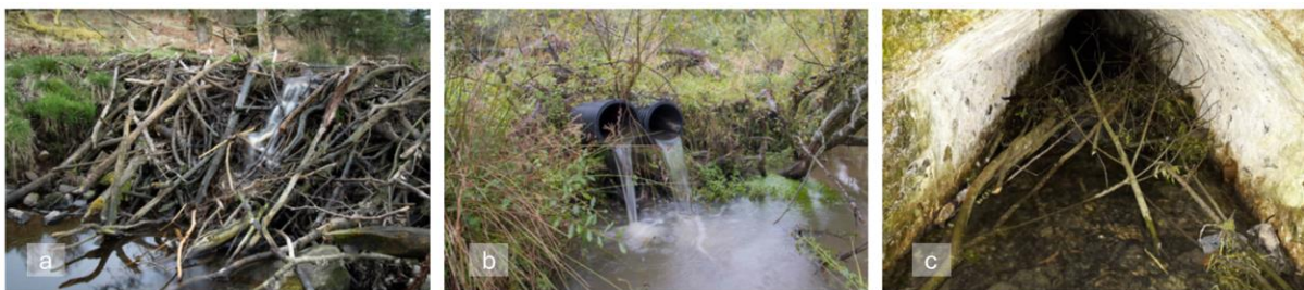
Figure 9. (a) Dam notching (b) Flow devices (c) Culvert protection. Beaver Management (2021).
