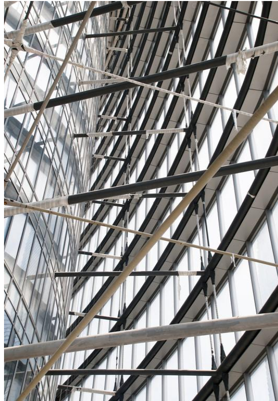
Figure 1.11: Picture of the cavity of double skin Façade of Shanghai Tower in China.
