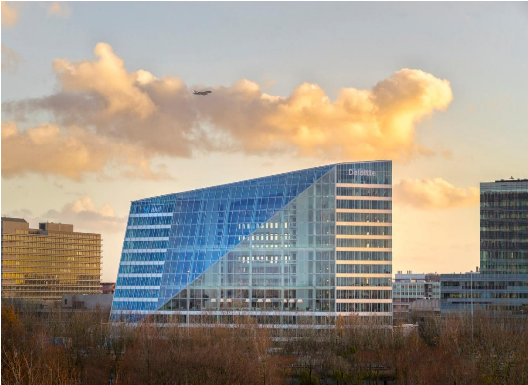
Figure 1.18: Northern façade of “The Edge”, Amsterdam, Netherlands.
