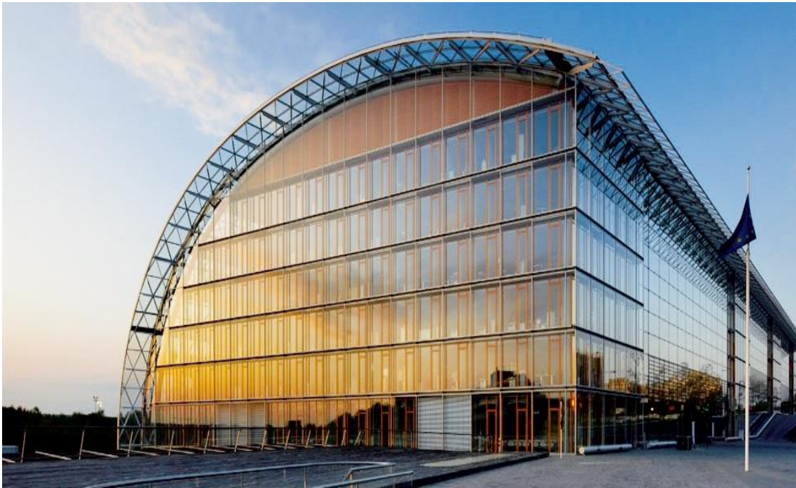
Figure 1.20: European Investment Bank Building completed in 2008 (Luxemburg).
