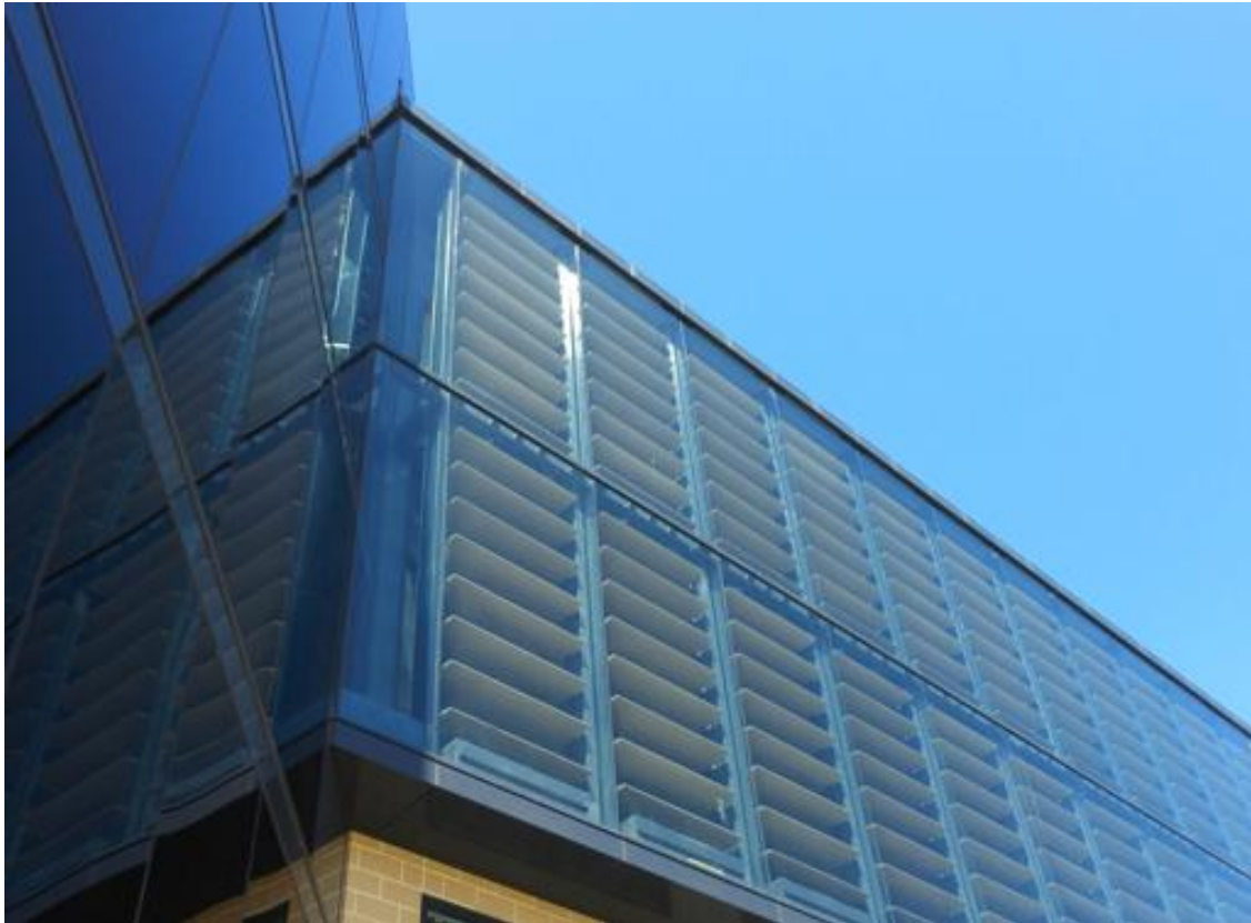
Figure 1.14: Example of shading inside the DSF cavity. Horizo Company, Australia.
