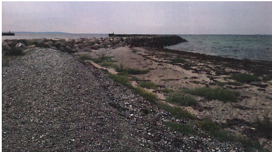
Figure 4.5: Area B, it can be seen the pebble berm close to the brakwater.
