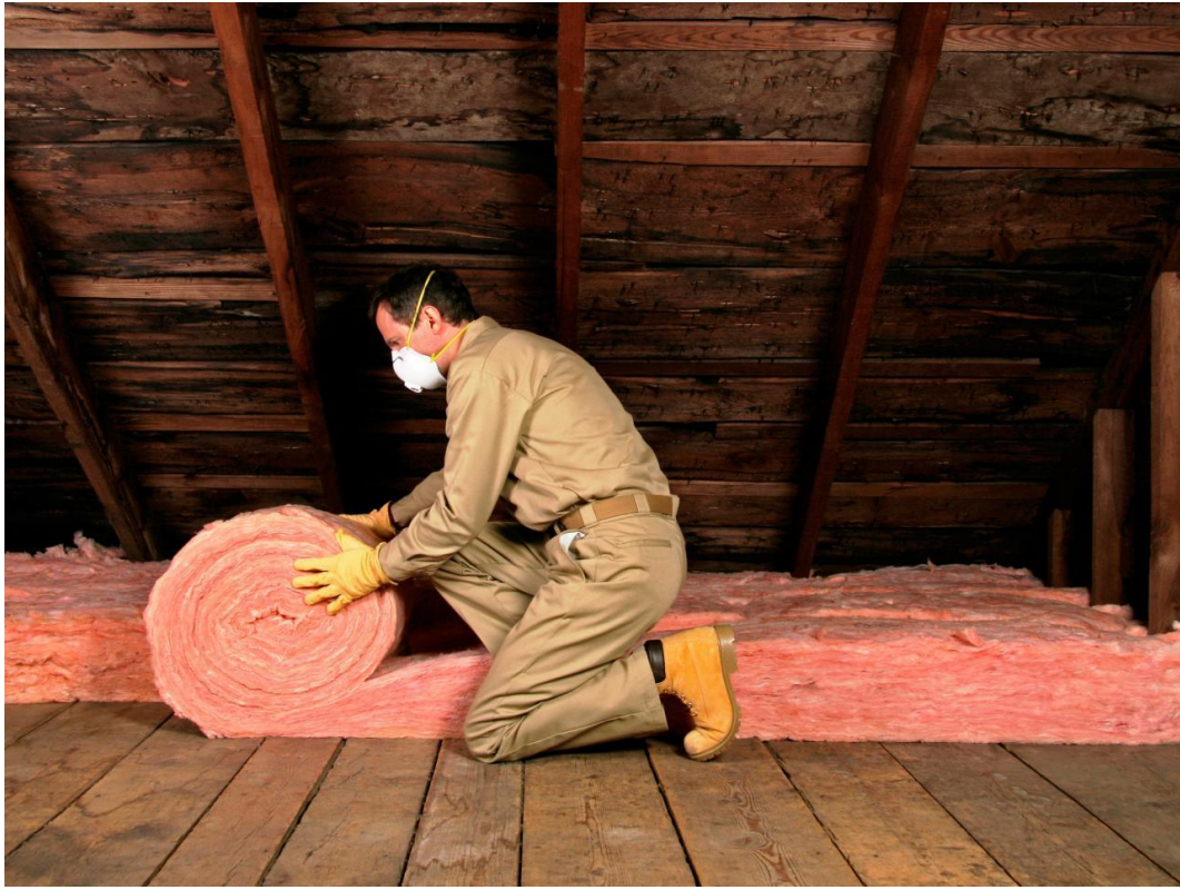
Figure 6.6 - Attic slab insulation
