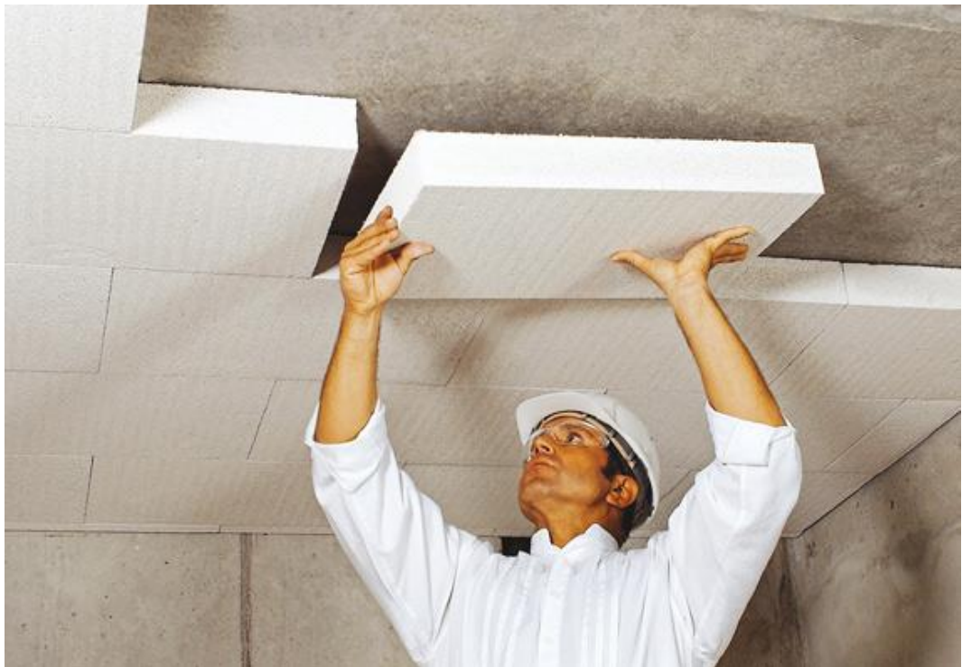
Figure 6.5 - Cellar slab insulation
