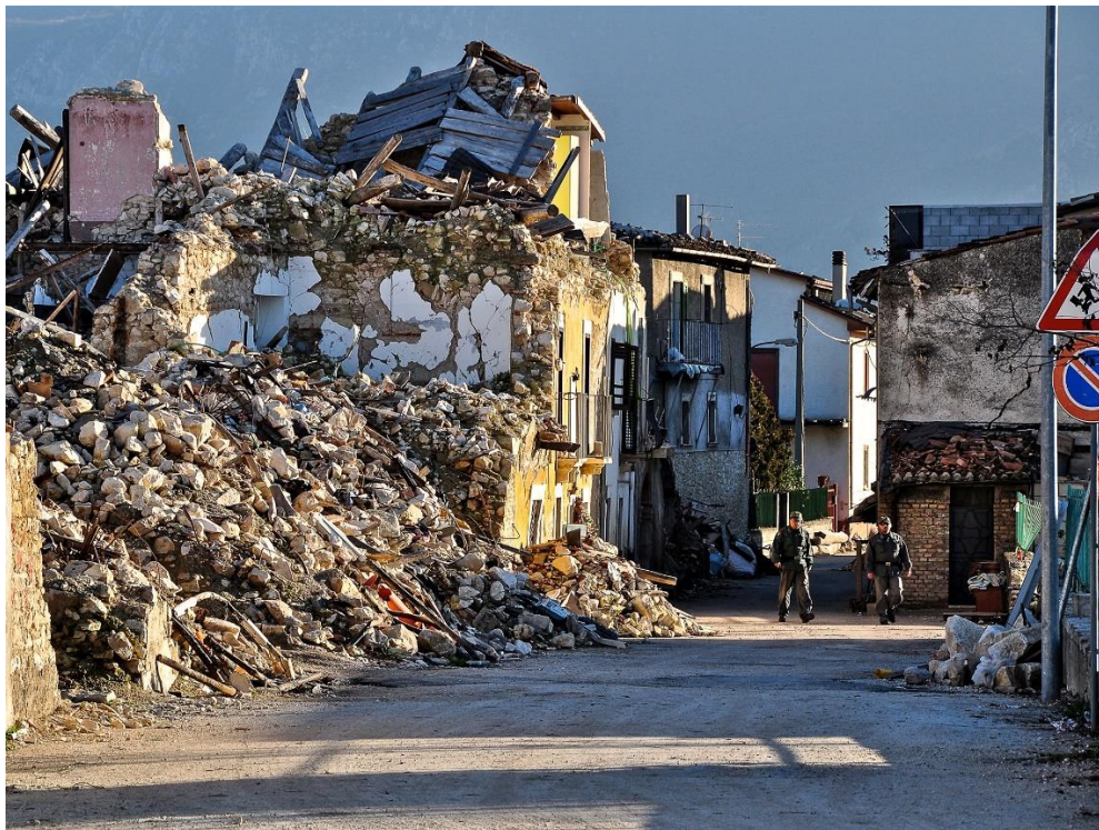
Figure 1 : L'Aquila Italy earthquake 2009
