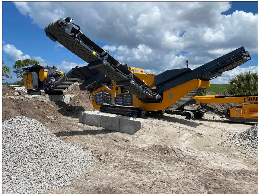
Figure 3 Screener used for sorting crushed concrete into different sizes.
