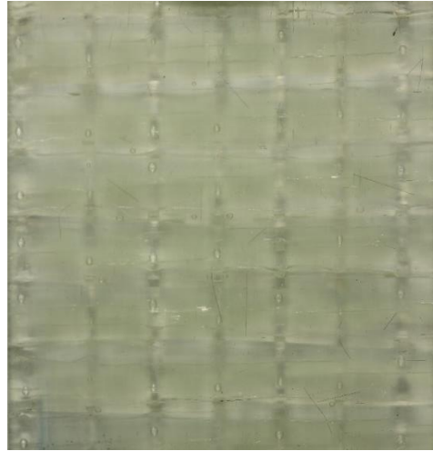
Figure 7.7: Photography of the damage that is visible in a specimen tested before failure
