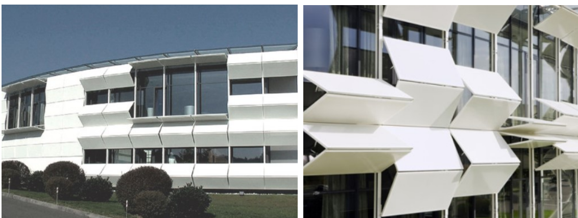
Figura 45:a- Facciata Kiefer Technic Showroom, Austria, 2007, tratto da Design approaches and typologies of adaptive facades: A review; b- Kiefer Technic Showroom dettaglio pannelli, 2007, tratto da Design approaches and typologies of adaptive facades: A review
