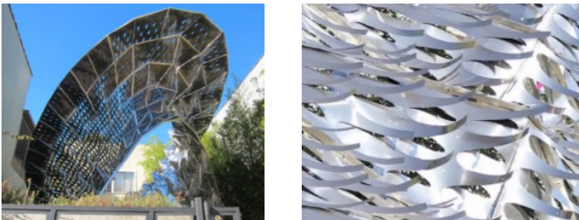
Figura 46:a- Foto facciata The Bloom, Los Angeles, 2012, tratto da Design approaches and typologies of adaptive facades: A review ; b- Dettaglio elementi di schermatura, tratto da Design approaches and typologies of adaptive facades: A review
