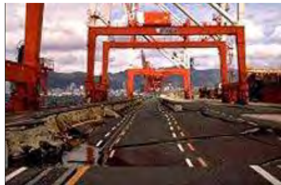
Figure 1.4 Highway damaged after the earthquake
