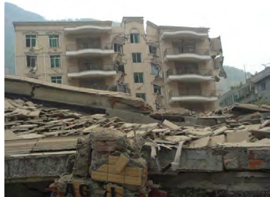
Figure 1.2 A bank in Beichuan after the earthquake
