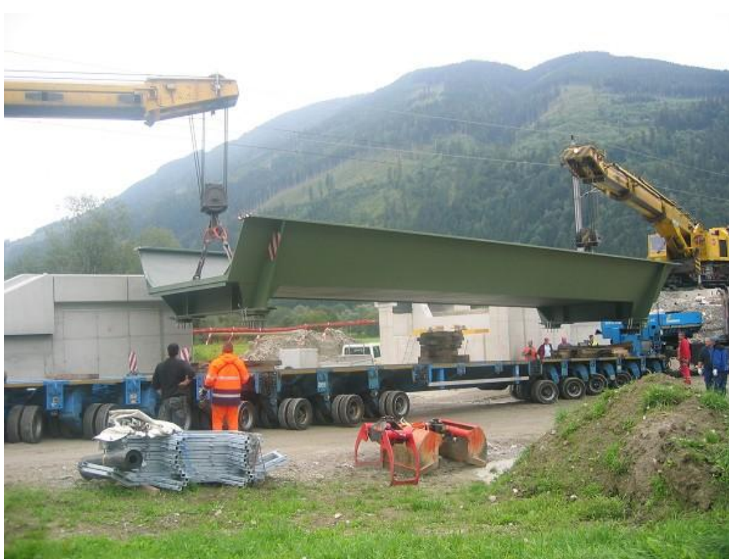
Figure 4 View of Eisenbahnbrücke Brunngraben bridge
