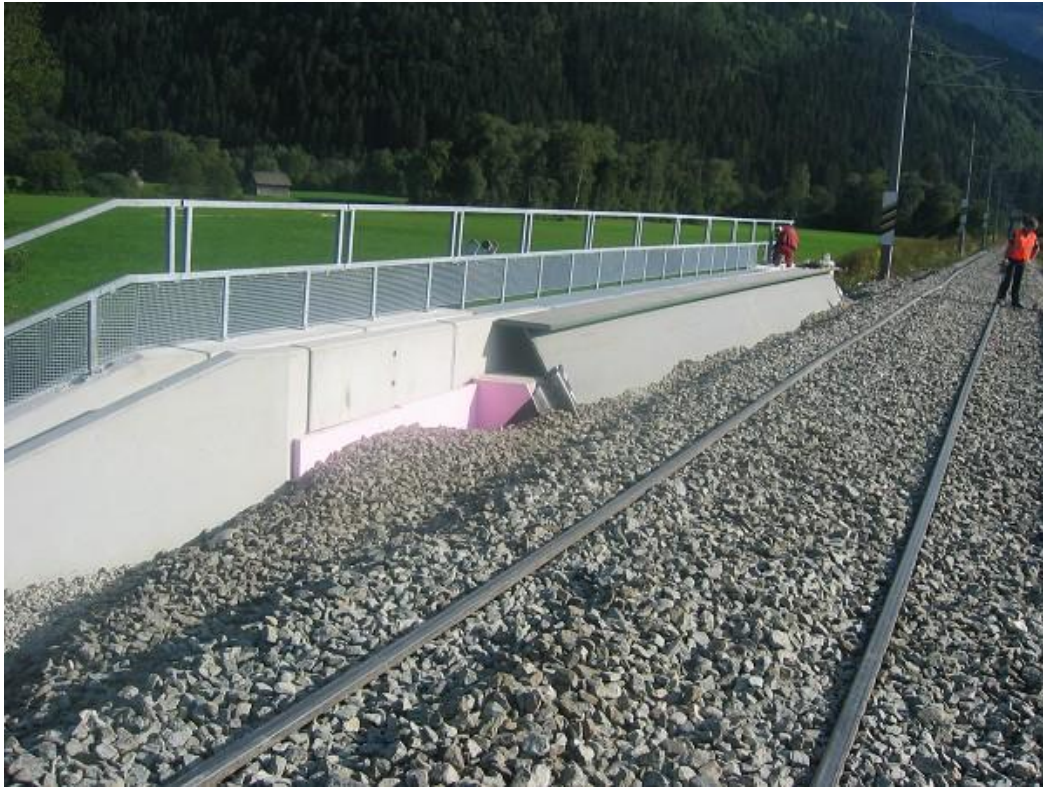
Figure 3 View of Eisenbahnbrücke Brunngraben bridge
