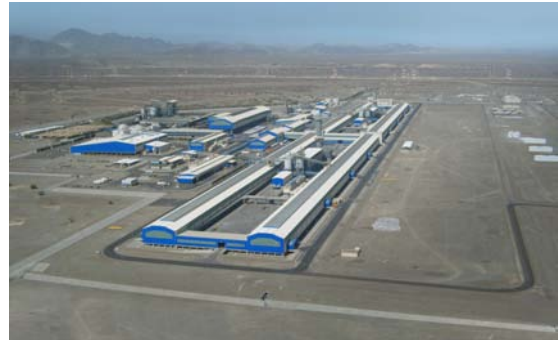
Figure 7.14: Example of Aluminium Smelter.
