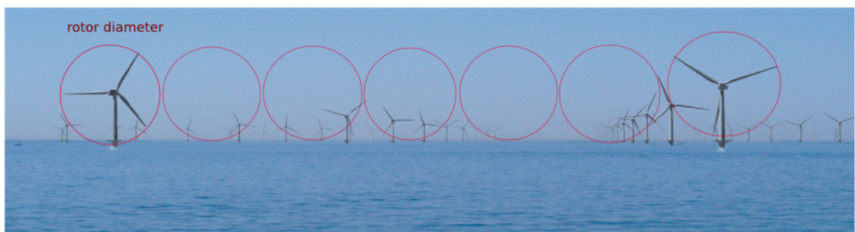
Figure 2.1. Proximity constraint. The red circles represent a rotor diameter: typically the minimum distance between turbines is around four or five rotor diameters.
