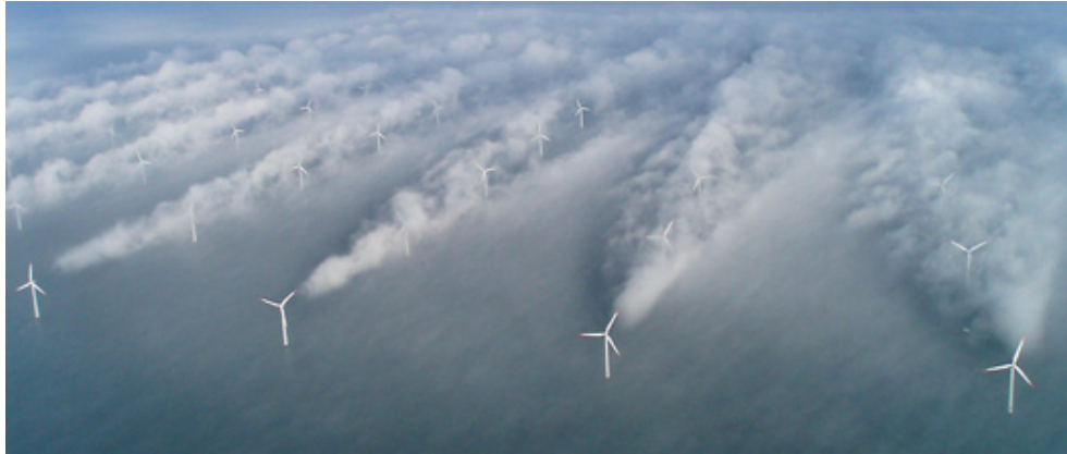
Figure 1.3. Wake effect in the Horns Rev 1 wind farm [2]
