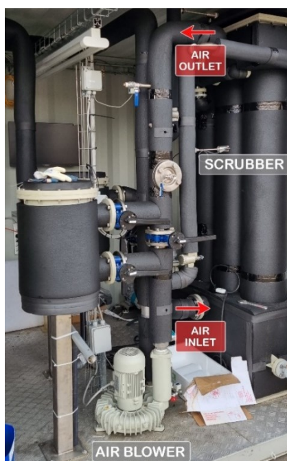
Figure 2.5: Absorption reactor (scrubber) and air flow path
