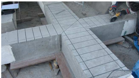
Figure 3.68 – Cutting grooves on the top surface
