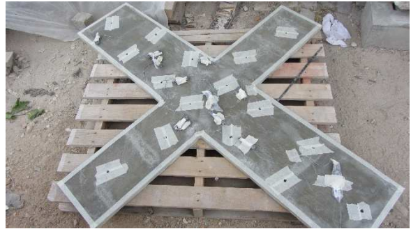
Figure 3.54 – Drilling of hole in the panel
