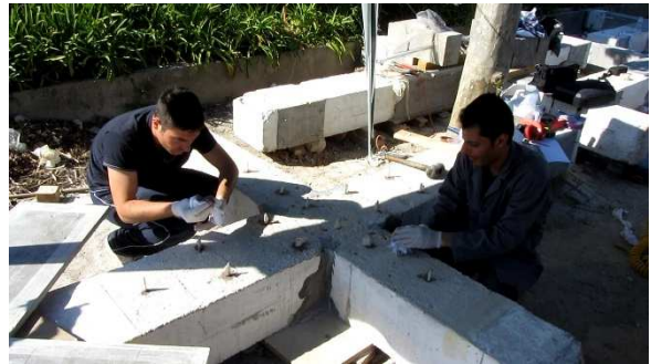
Figure 3.42 – Putting the anchors
