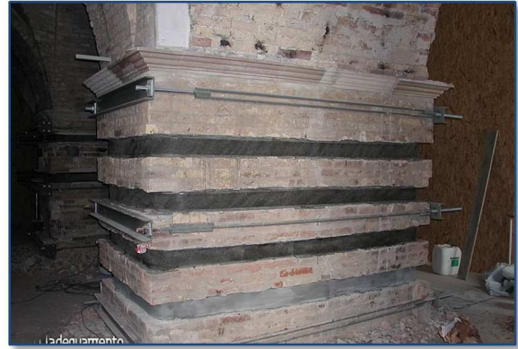
Figure 2.4 – Externally bonded FRP on masonry columns
