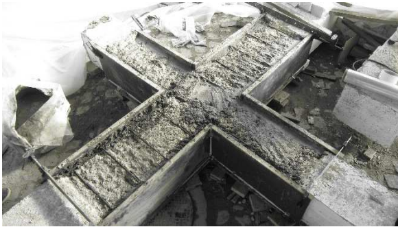
Figure 3.75 – Casting of normal concrete
