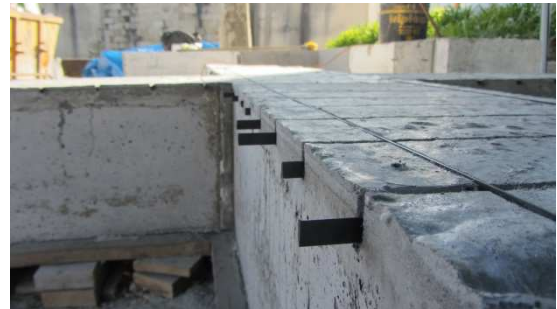
Figure 3.30 – intersection between carbon laminates
