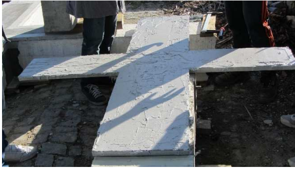
Figure 3.57 – Spreading of glue in the panel
