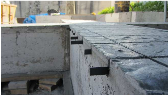
Figure 3.81 – View 1 of CFRP bars into the groove
