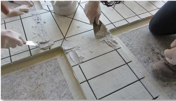
Figure 3.21 – Filling grooves with epoxy glue
