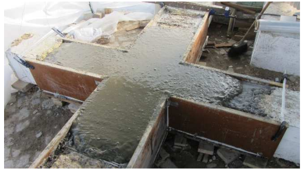
Figure 3.76 – Casting of SHCC
