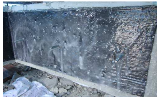
Figure 3.60 - Spreading of epoxy glue on the panel
