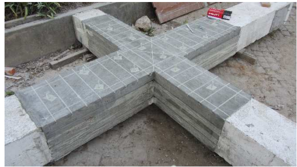
Figure 3.73 – Putting of anchors in JPB
