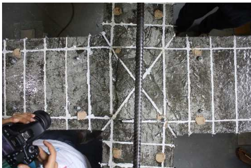
Figure 4.16 – Crack on the top surface, JPA-3
