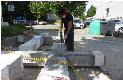
Figure 3.83 – Drilling the hole on the top surface
