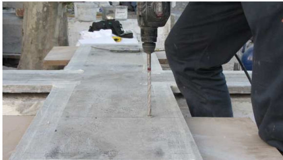
Figure 3.41 – Drilling panel
