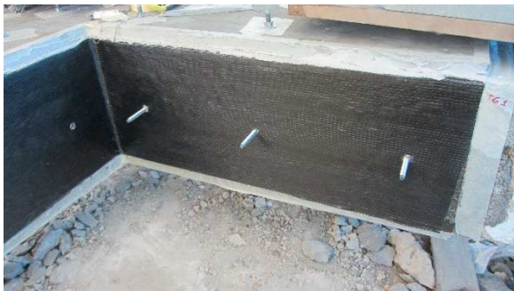
Figure 3.55 – Putting of the strain gauges
