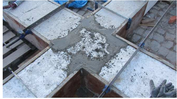
Figure 3.36 – Leveling of the surface
