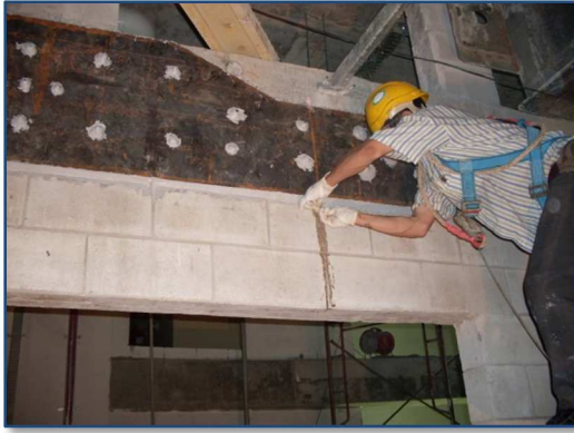
Figure 2.1 – External steel plate [7]
