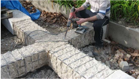
Figure 3.47 – Concrete removal
