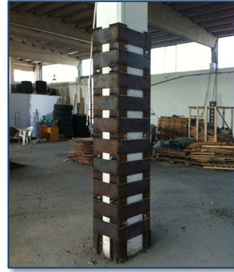
Figure 2.2 – Steel jackets [7]
