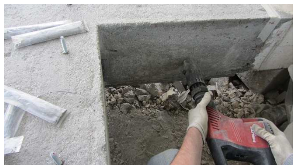
Figure 3.52 - Lateral surface roughened
