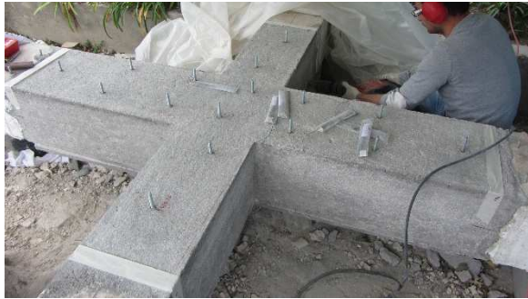
Figure 3.53 – Putting the anchors on top surface
