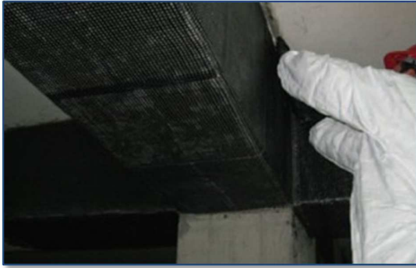
Figure 2.3 - Externally bonded FRP concrete columns
