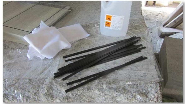
Figure 3.22 – Cleaning of carbon FRP laminates
