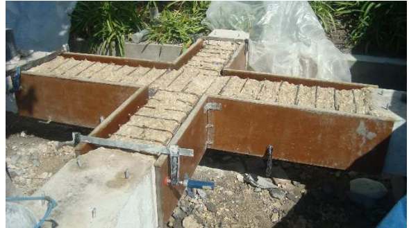
Figure 3.48 – Application of the formwork
