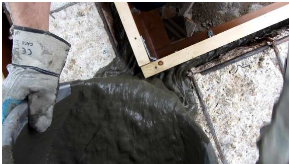
Figure 3.66- Casting SHCC material
