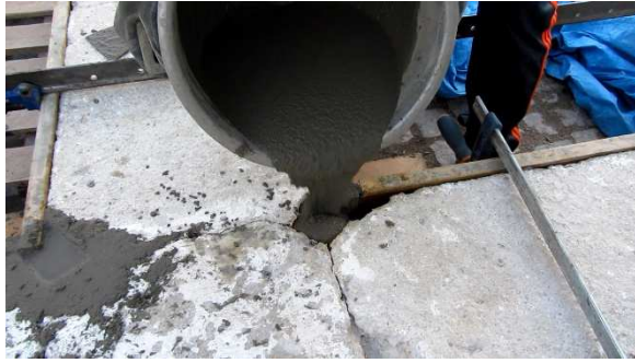
Figure 3.35 – Casting corner
