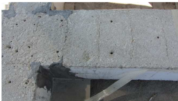
Figure 3.39 – Surface roughened
