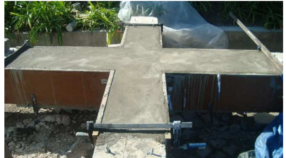
Figure 3.50 – Casting of the new concrete
