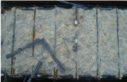
Figure 3.49 – Application of the strain gauges
