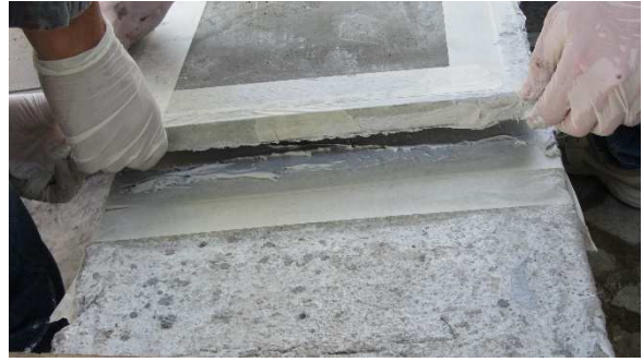
Figure 3.58 – Installation of the panel
