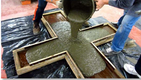
Figure 3.17 - Casting SHCC for precast panels
