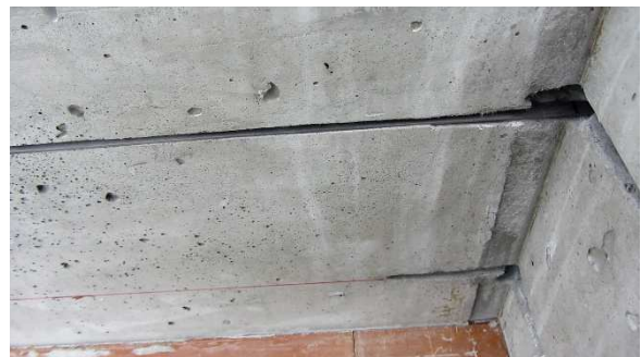
Figure 3.69 – Cutting grooves on the lateral surface
