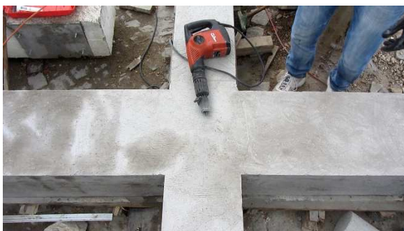
Figure 3.51 – Top surface roughened
