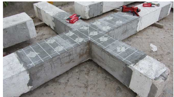
Figure 3.84 – Putting the anchors on JPA-3
