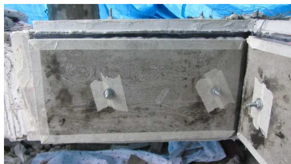
Figure 3.62 – Lateral strengthening completed
