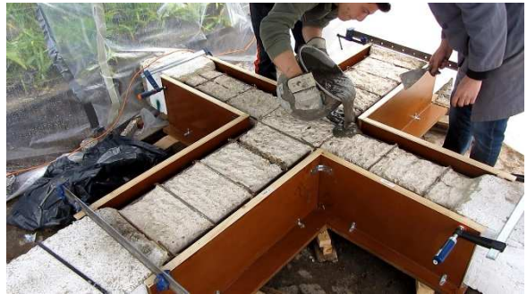
Figure 3.65 – Casting SHCC material
