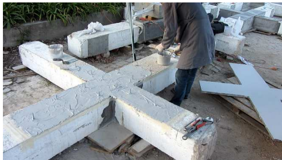
Figure 3.43 – Spreading of the glue
