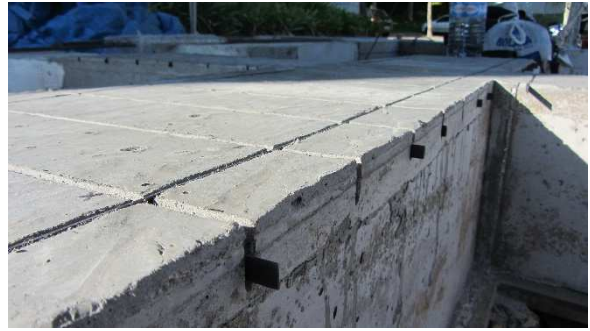
Figure 3.82 - View 2 of CFRP bars into the groove
