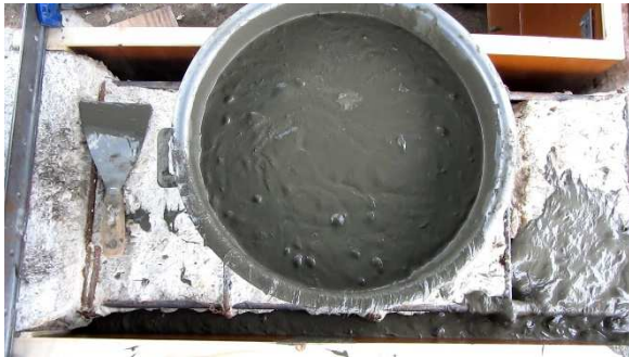
Figure 3.64 – Preparation of the mix
