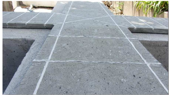
Figure 3.24 – Roughened surface ready
