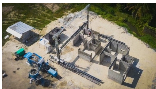
Figura 13. Stampante gantry-based (BOD3) [11].
