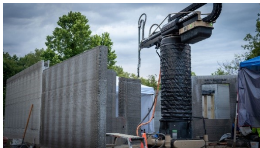
Figura 12. Stampante robotic-based (Frank) [10].
