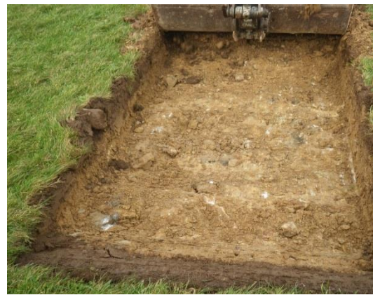
Figure 3.3 CSM: view of the first two layers.
