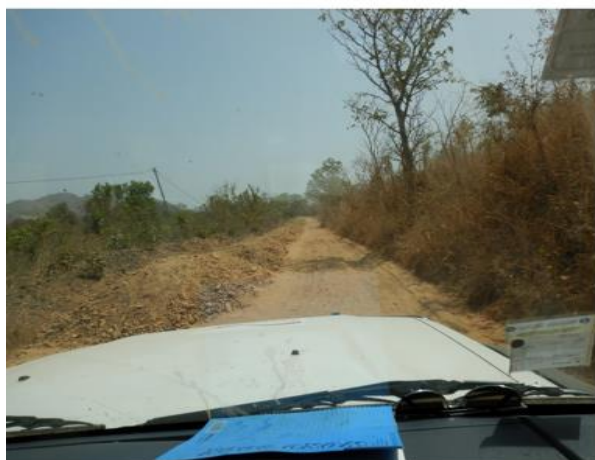
Poor road's network
