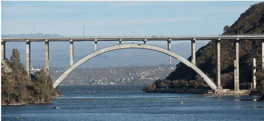
**Figure 1.18.** Spandrels of a deck arch bridge (midasbridge.com)
