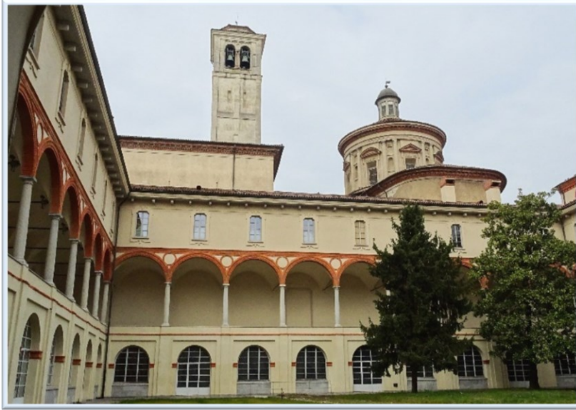
Fig. 2C. Interior of one of the two cloisters. Photo by L. MERY.
