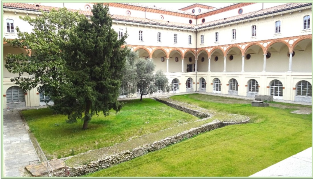
Fig. 2B-1. Interior of one of the two cloisters. Photo by L. MERY.
