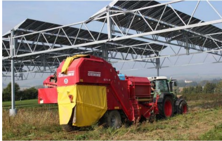
Picture 7 Overhead system enabling cultivation with a potato harvester (farm community Heggelbac, © Fraunhofer ISE).
