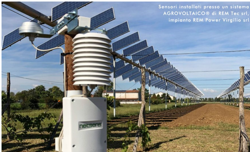
Picture 27 Sensors for monitoring in agrivoltaic systems (© Netsens-RemTec)
