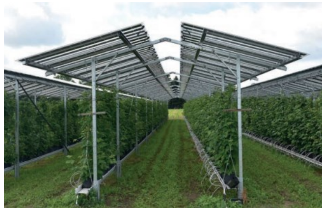
Picture 5 Overhead system for orchards (© BayWa r.e.)
