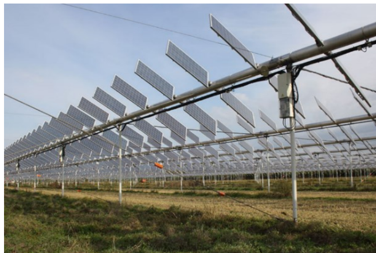
Picture 6 Advance APV system with dual axis tracker (© https://remtec.energy/ )
