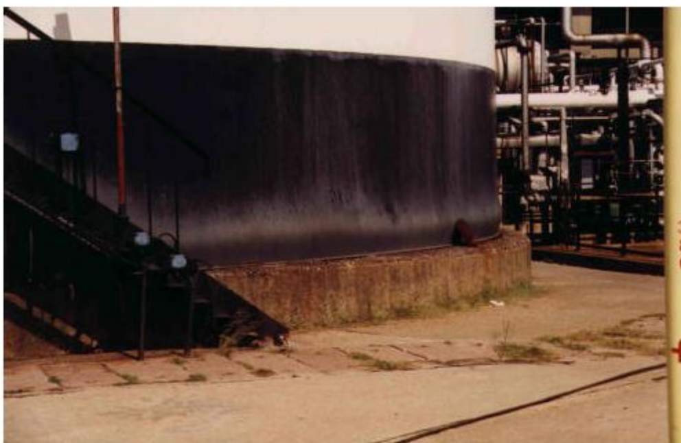
Fig.3.2-Elephant foot buckling non severo
