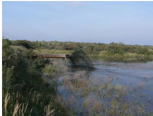
Figure 7: Dredged material pumped onto a spoil field
