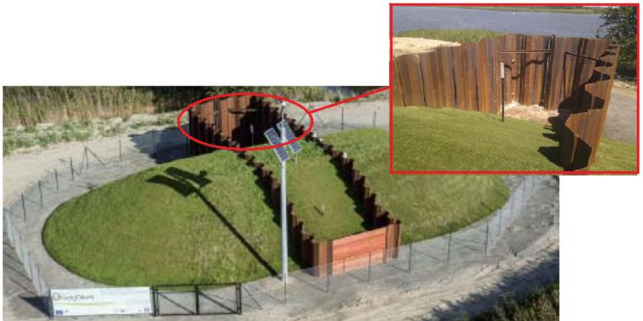
Figure 11: Test dikes and sheet-pile wall
