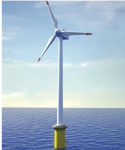
Figure 5. Monopile foundation of offshore wind Turbine [24]
