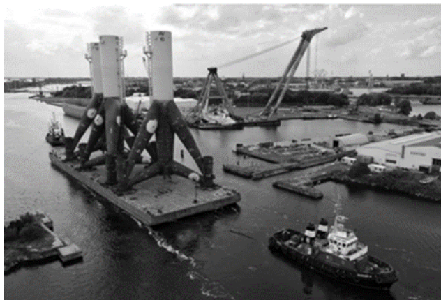
Figure 6. Tripod on a barge, on their way to Alpha Ventus wind farm [25]
