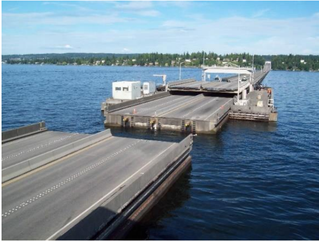
Figure 1.24. Retractable bridge (Google Search, 2022)
