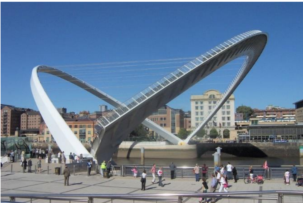
Figure 1.5. Gateshead Millennium Bridge (Google Search, 2022)
