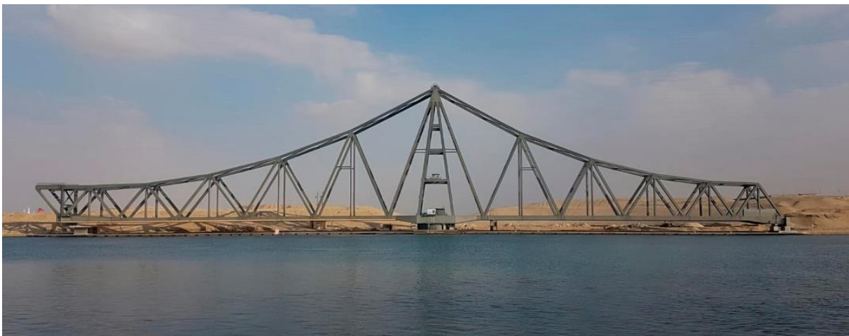
Figure 1.20. Swing bridge (Florida Department of Transportation, 2018)
