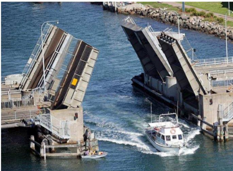
Figure 1.6. Bascule bridge (Florida Department of Transportation, 2018)
