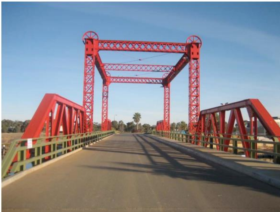
Figure 1.15. Vertical lift bridge (Florida Department of Transportation, 2018)
